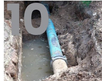
10 PIPE BACK TO SERVICE
