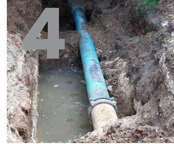
4 SURVEY TO ASSESS PIPE CONDITION & ABNORMALITIES
