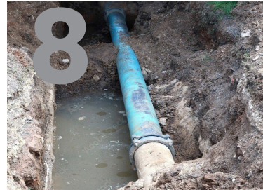
8 SURVEY TO CONFIRM LINING INTEGRITY
