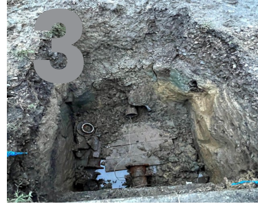
3 ISOLATE & CUT INTO THE PIPE
