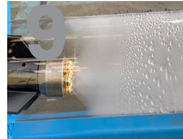
9 DISINFECT THE PIPE
