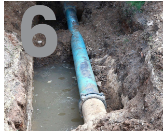
6 SURVEY TO CONFIRM PIPE IS CLEAN
