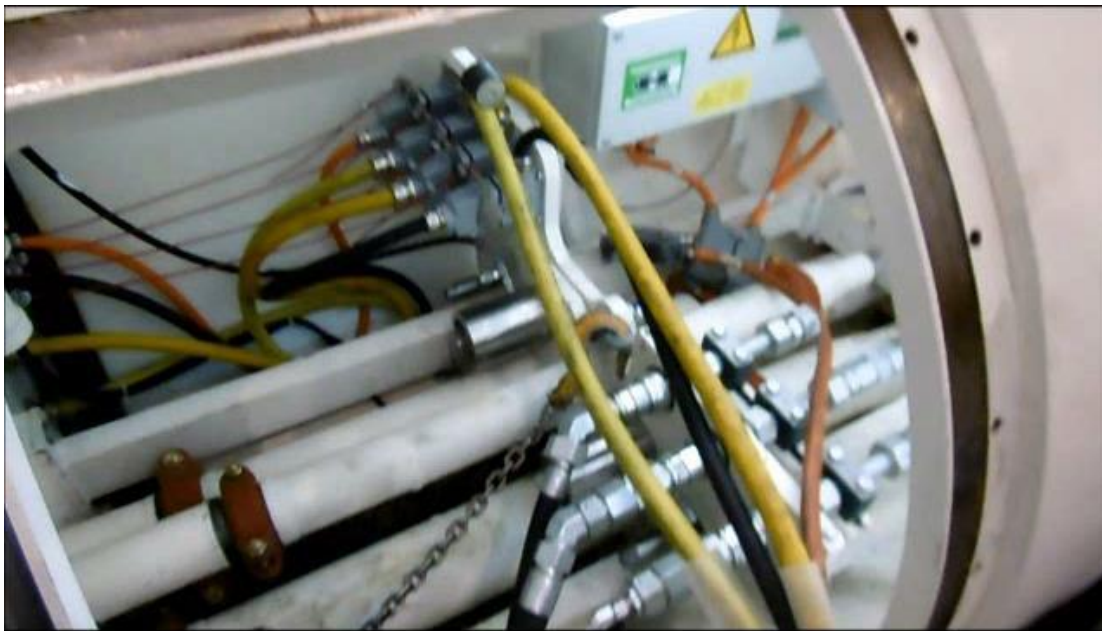
Direct Pipe®: remote disconnection for marine outfall
